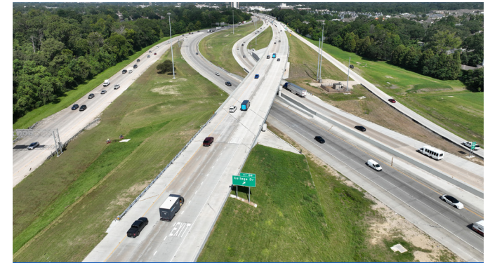
GEC maintained 3 lanes of traffic on I-12 WB and 2 lanes on I-10 WB throughout construction on a highly-congested interstate segment in Baton Rouge
