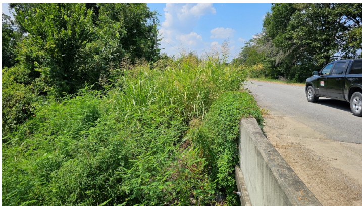
Figure 3-15: Example of In-accessible structure
