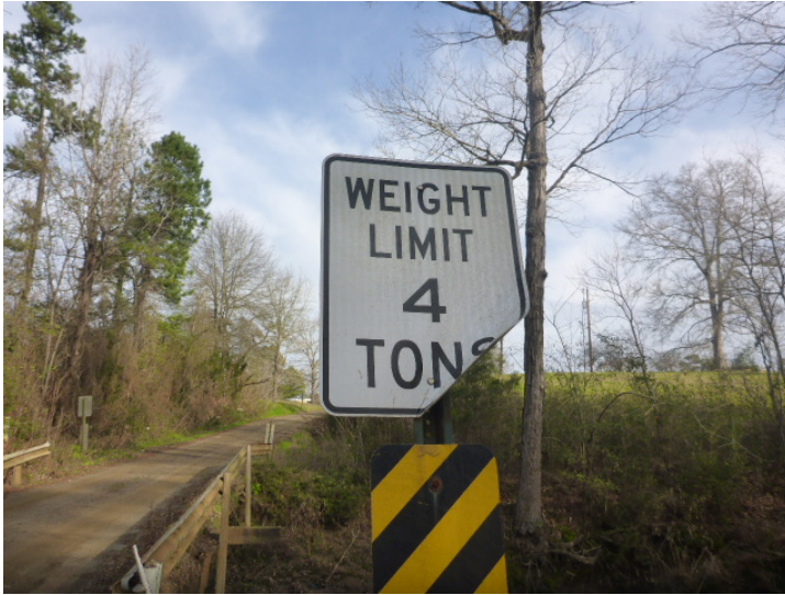
Figure 3-11: Damaged and incorrect weight limit sign
