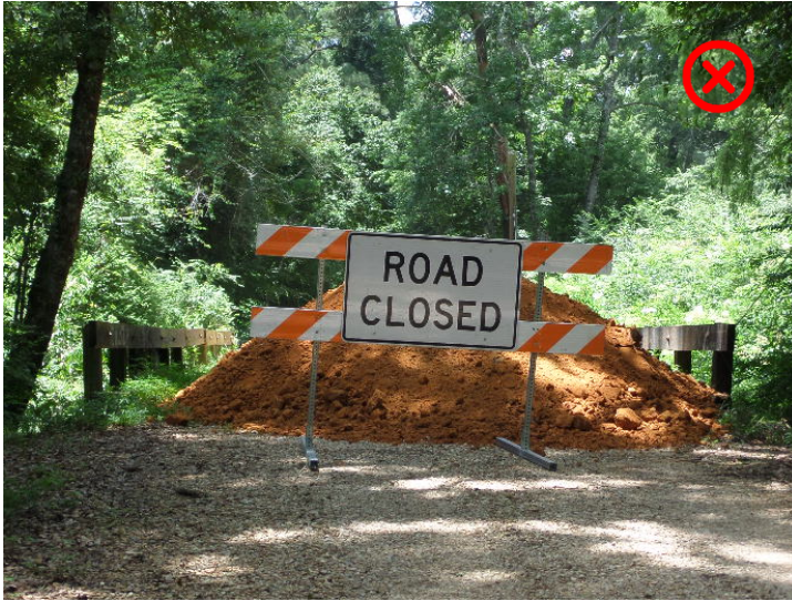
Figure 3-7: Incorrect closure using dirt pile
