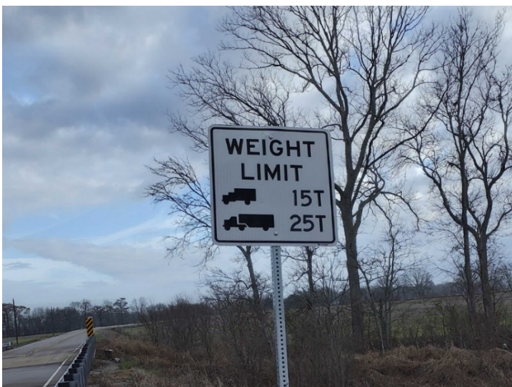
Figure 3-10: Correct weight limit sign
