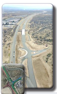
Project Description This \$34 M CMAR project involved reconstruction of 7-miles of 2-lane SR260 roadway into a divided 4-lane highway. A major component of the project was design of seven modern multi-lane roundabout intersections instead of signals to accommodate planned development along the corridor. The project included a new bridge, rehabilitation of the existing highway bridge and reconstruction of numerous box culverts.
