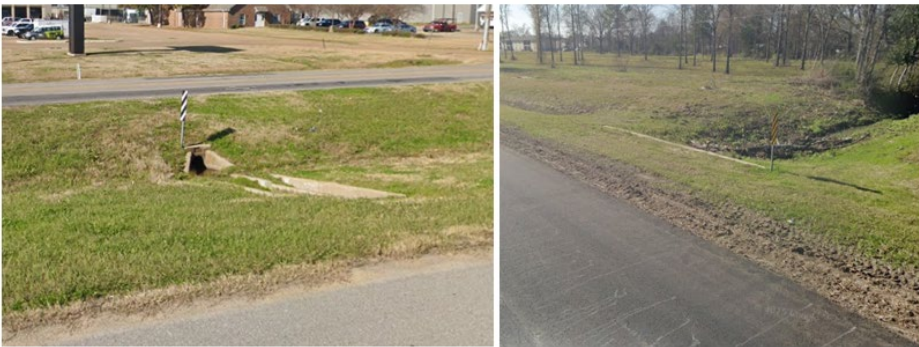
Figure – Existing drainage structures impacted by proposed bulb-outs
