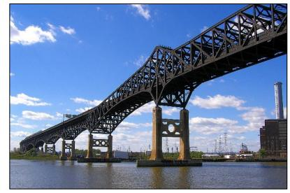
systems. The project consists of removal of the existing coating system (potential lead abatement), recoating of the structure (cleaning and painting), bridge structural repairs, deck patching, deck joint repairs, structural concrete patching, navigation clearance gauge replacement, and electrical system work including aerial beacon and navigation light system replacement.
