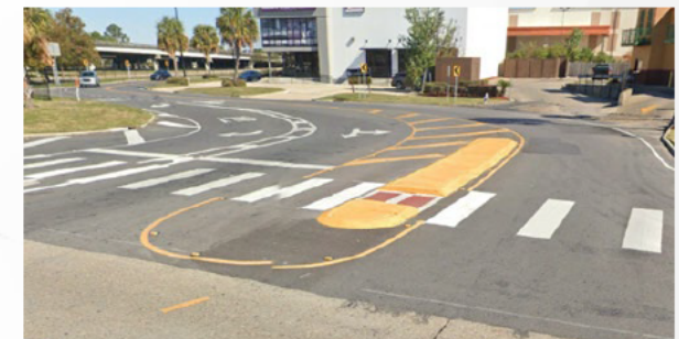
Figure: High visibility crosswalk and pedestrian refuge installed at I-10 Service Road and Read Boulevard
