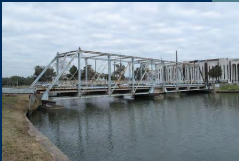
MAGNOLIA PEDESTRIAN BRIDGE BEFORE & AFTER
