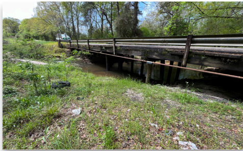
Photo showing channel meandering near southern abutment (3/26/2024)
