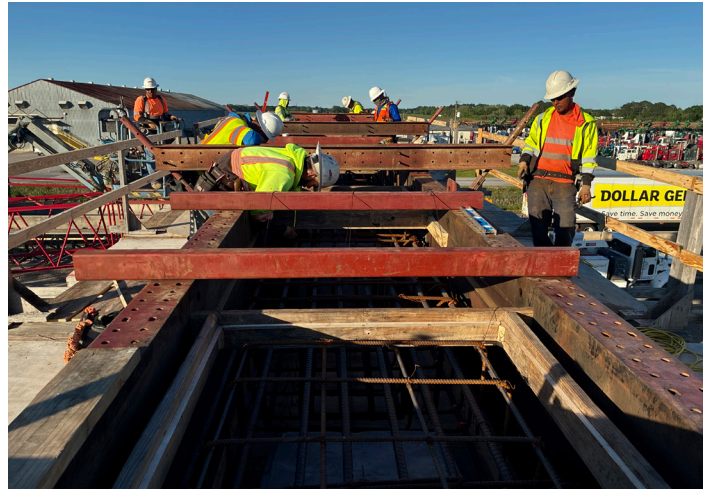
Installing caps on the U.S. 90 railroad overpass in Iberia Parish
