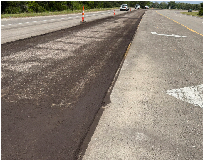
Milling on LA 27 in Calcasieu Parish
