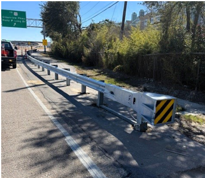
Completed Clearview Parkway guardrail repairs in Jefferson Parish
