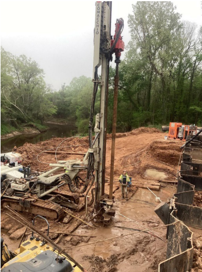
LA 454 Wiggins Bayou Bridge in Avoyelles Parish
