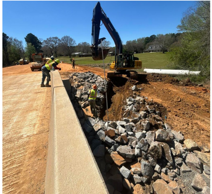
LA 818 bridge replacements in Ouachita Parish
