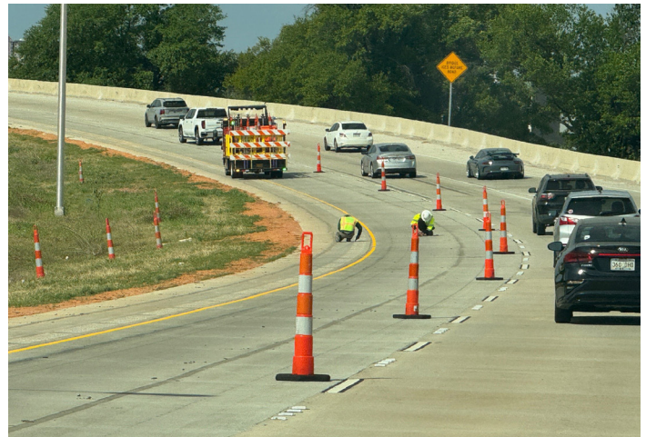
Striping on the I-20 rehab project in Bossier and Caddo parishes
