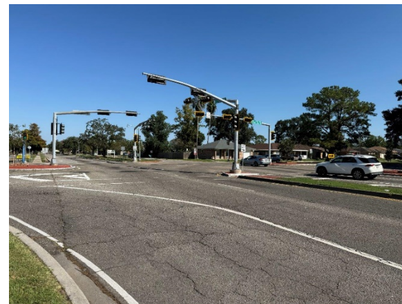
Loyola Drive at West Loyola Drive
