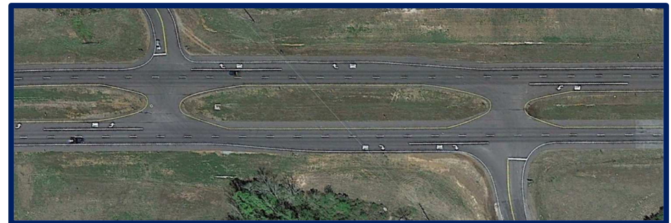
Figure18.1 - 417-01-0015 / LA 28 (LA 121 to LA 465): Vernon Parish (2008)
