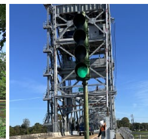
Jackson St Lift Bridge
