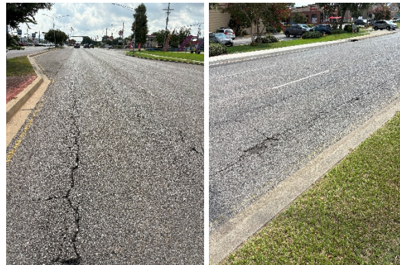
Figure 1: Asphalt Deterioration
