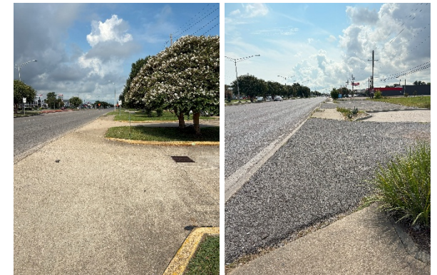
Figure 2: Driveways/Detectable Warning Surface Locations
