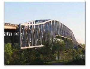
The Krotz Springs Bridge is owned and operated by LADOTD. The bridge was constructed in 1973 and consists of eastbound and westbound structures. Each bridge carries two lanes of vehicle traffic over the Atchafalaya River in Krotz Springs, Louisiana. The bridges consist of a three-span truss main span that
