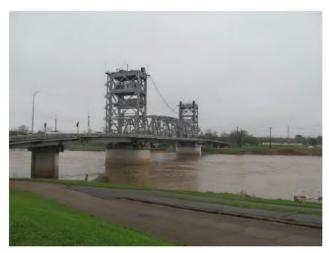
The Jackson Street (Red River) Lift Bridge in Alexandria, Louisiana, carries two lanes of traffic over the Red River. The main span is a through truss design with a 300' vertical lift span centered between the two towers.
