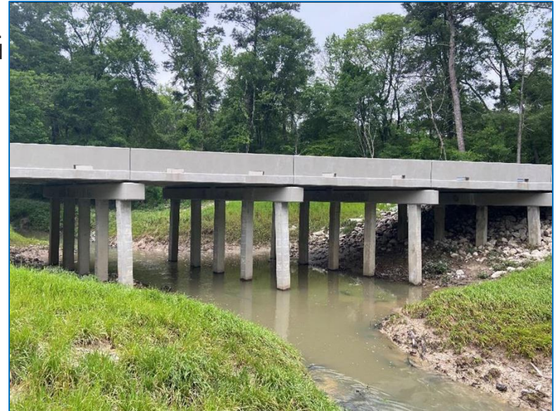
Whittington Road Bridge over Grays Creek
