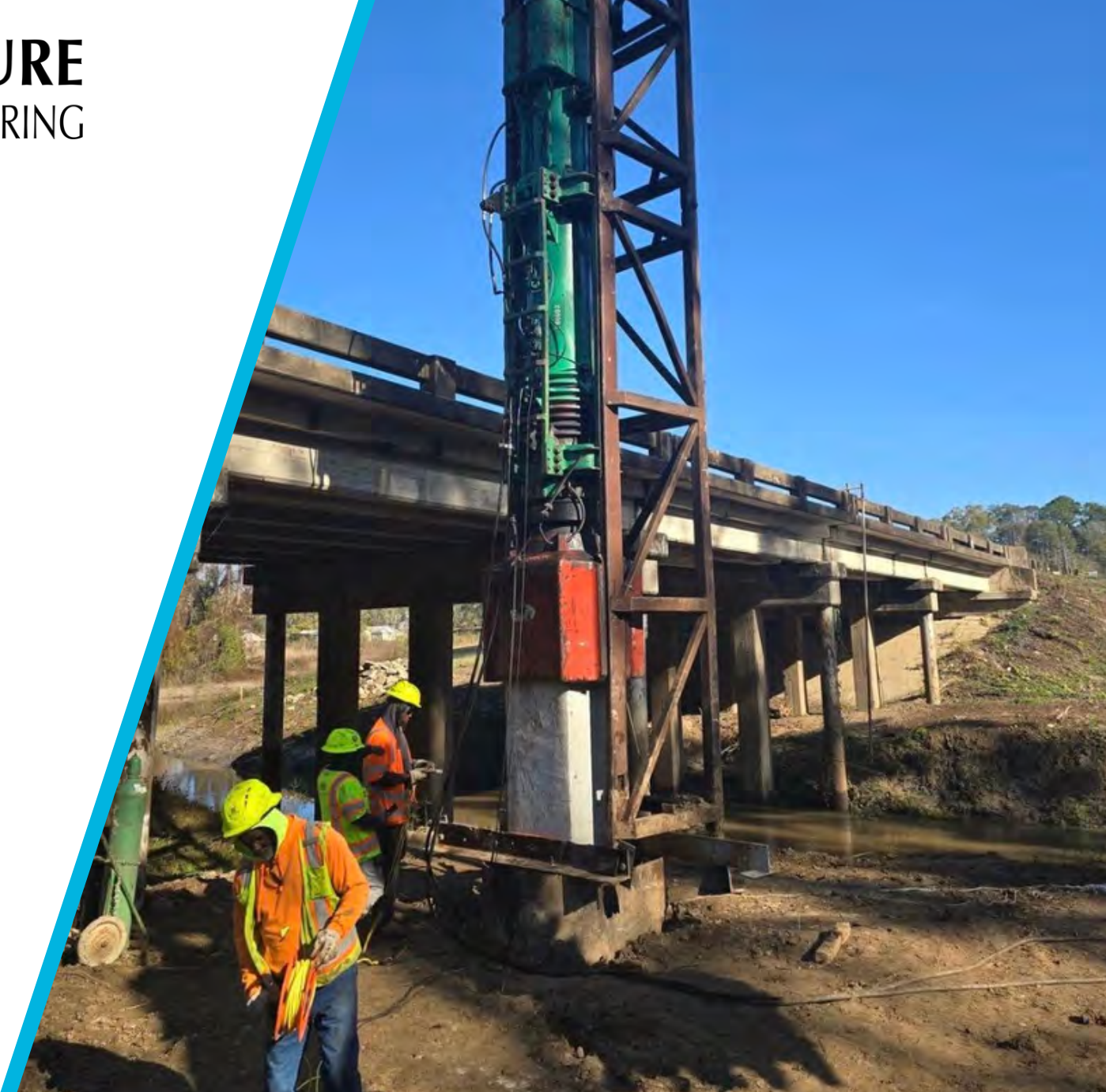
Bayon Carron Bridge Project -Bridge Foundation Construction
