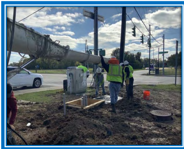
Signal Foundation Installation : Lafayette, LA
