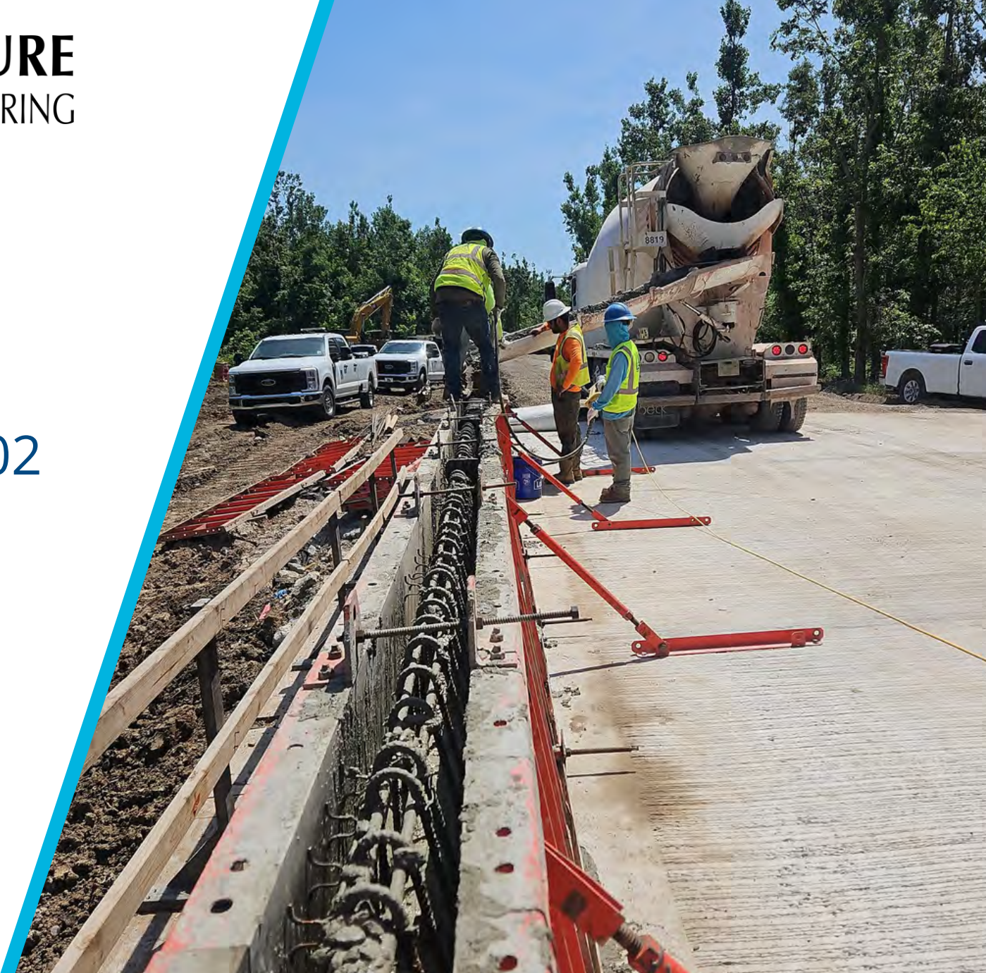
US 90 RR Overpass Project
