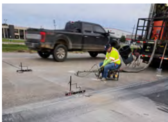
US 90 construction operations: slab jacking (left) and asphalt overlay (right).
