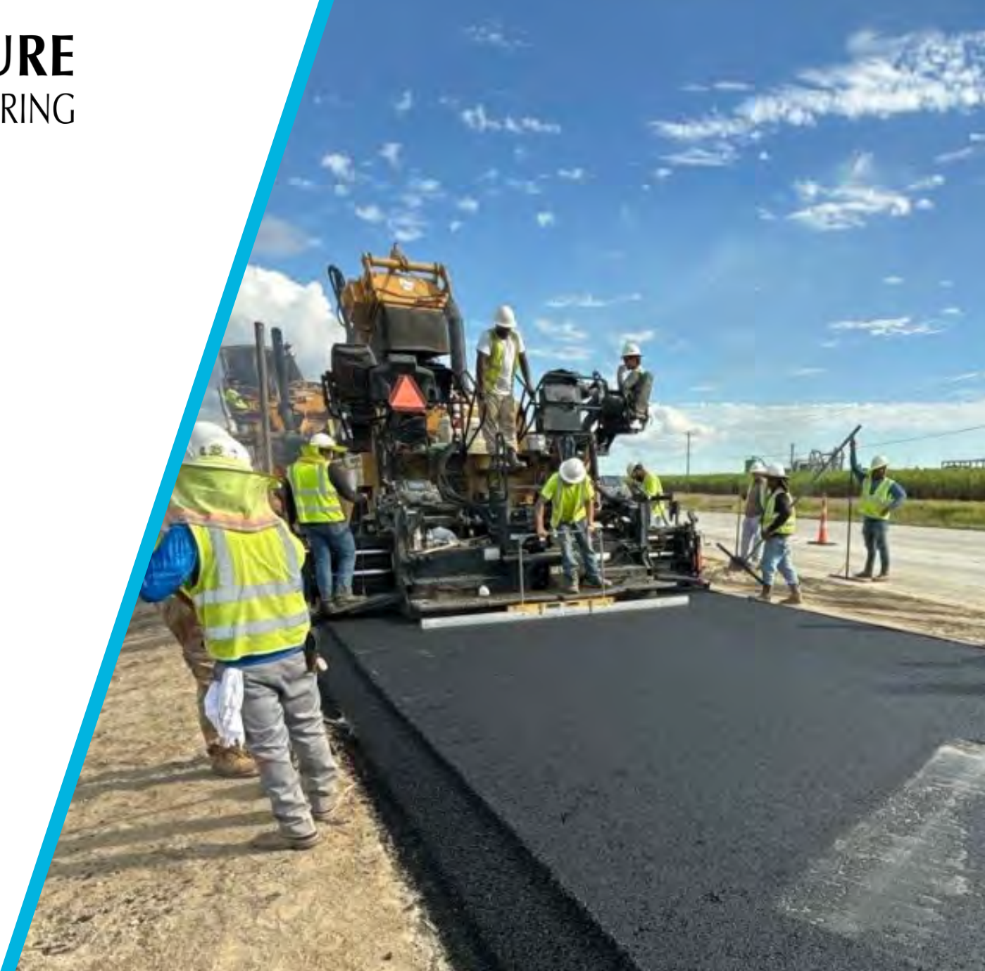
US 90 RR Overpass Project - Asphalt Paving Operations
