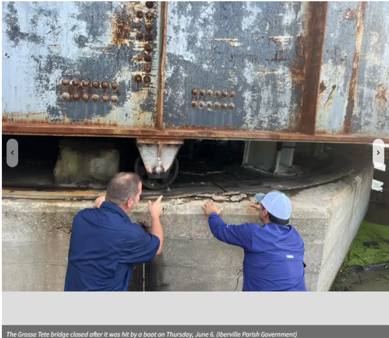
Figure 7: Inspecting concrete and pivot pier damage.
