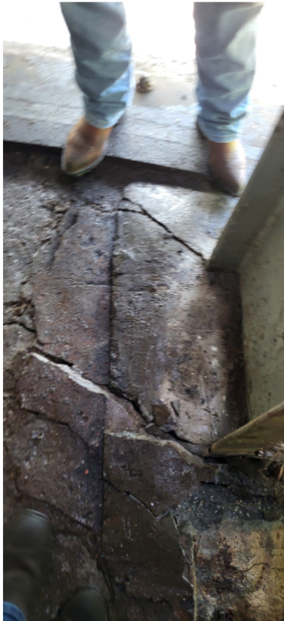
Figure 6: Concrete damage pivot pier cap.
