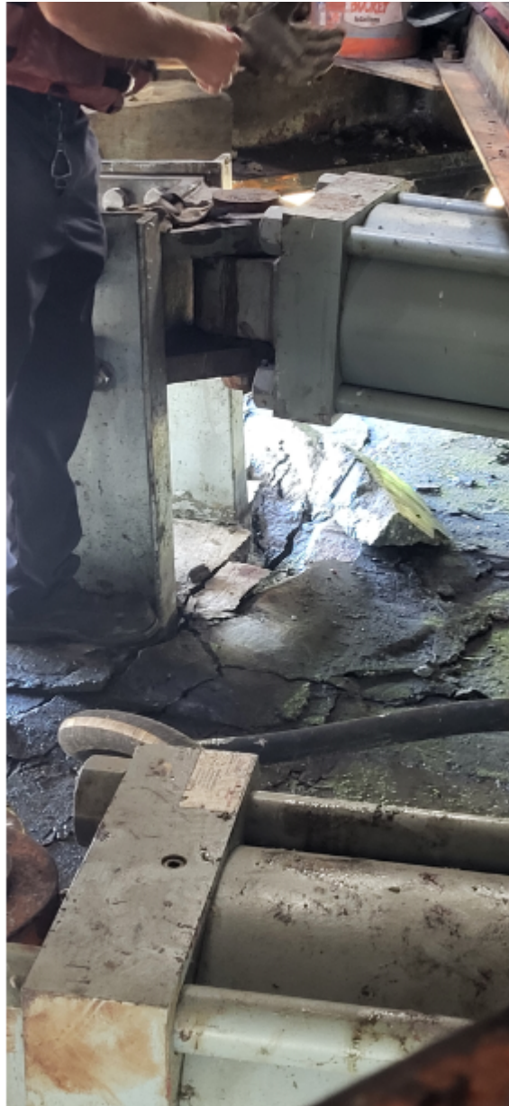
Figure 3: Pivot pier damage.
