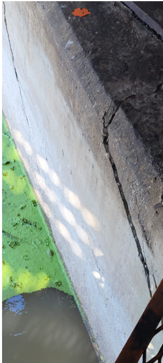
Figure 4: Concrete structure damage of pivot pier.
