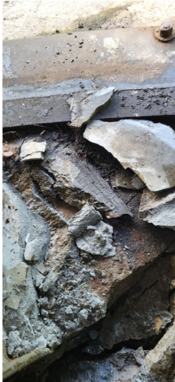
Figure 5: Close up of concrete and structural damage.
