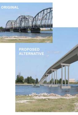
Both movable- and fixed-span designs were considered along with three preliminary alignments. LADOTD Design Guidelines and EDSMs along with the LADOTD Road Design and Bridge Design Manuals were utilized.
