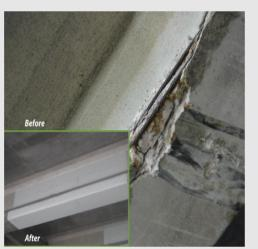
the prestressed concrete bridge beams, damaging six of the beams on the third span of the bridge. Northbound Regal Row was shut down due to the risk of falling debris. The preliminary, emergency field report revealed no serious structural damage to the bridge and northbound Regal Row was reopened to traffic. A **close collaboration with the contractor enabled the repairs to be completed three days** after the issuance of the final signed and sealed bridge repair plans.
