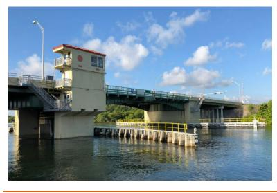
To improve bicycle and pedestrian safety, the sidewalk grating was replaced with aluminum plates, guardrails and curbs were improved at the east and west transitions, and new bicycle friendly plates were added in the shoulders. To facilitate maintenance and inspection, the project includes the addition of new inspection/maintenance stairs and platforms to bascule piers/traffic gates/equipment, and upgrades to the control house.
