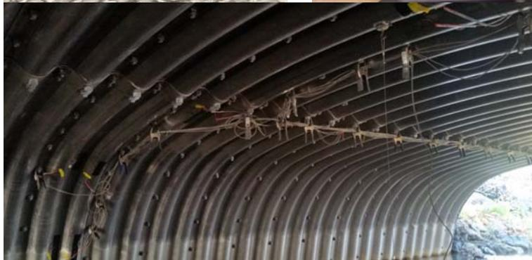
**Figure 24 – M6C2 Culvert Instrumentation**
