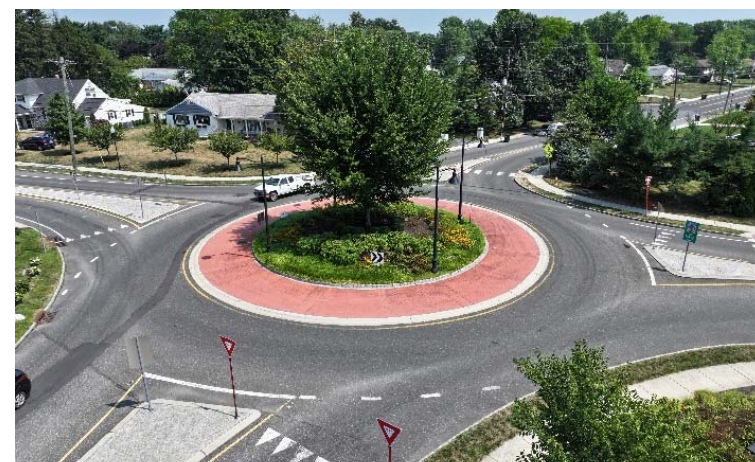
BH PROJECT Riverton Road Traffic Circle
