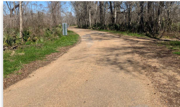
Photo taken from Spring Bayou bridge showing horizontal geometry without superelevation
