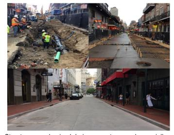
prevention. The main causes of flooding on Bourbon Street were undersized drainage systems and especially, the clogging or collapsing of existing drain lines due to directional boring utilities and large amounts of littering and debris. By maintaining a sustainability and environmentally conscious mindset, Mott MacDonald proactively designed adequate drain line sizes and new curb-guards on the stormwater inlets to vastly reduce the ability of litter to enter the new stormwater drainage system.
