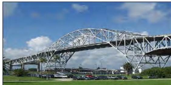
Corpus Christi Harbor Bridge, a Through Truss and Deck Truss Structure, is 1782 feet in Length
