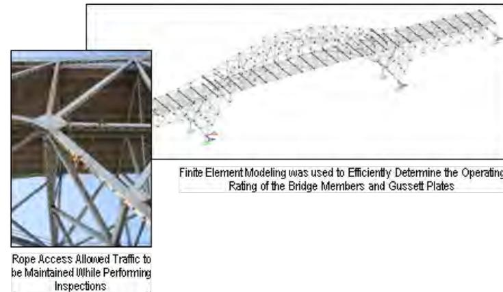
Finite Element Modeling was used to Efficiently Determine the Operating Rating of the Bridge Members and Gusset Plates
