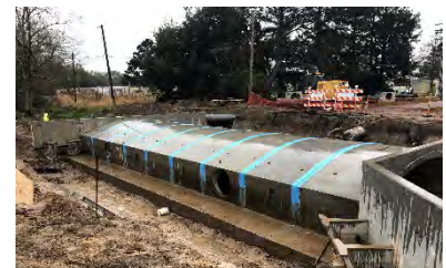
Conspan bridge during construction
