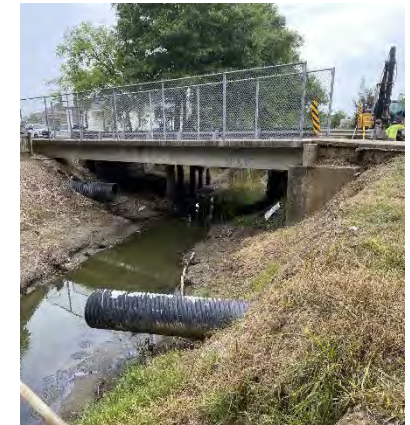
Existing East Martial Ave Bridge to be replaced
