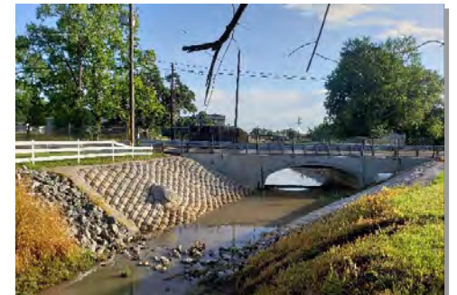
Completed conspan bridge
