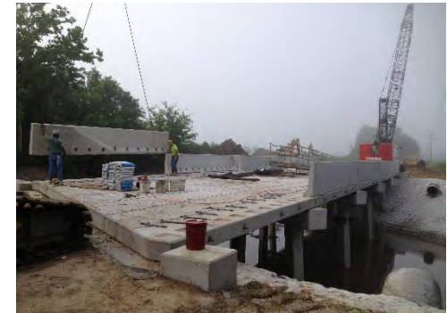
Bridge during construction
