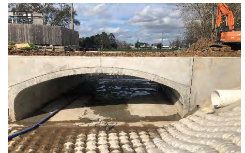
Completed conspan bridge
