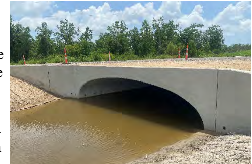
Completed conspan structure
