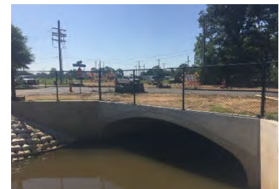
Completed conspan bridge
