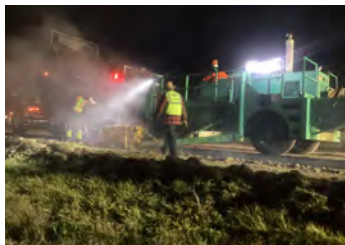
US 90 construction operations: slab jacking (left) and asphalt overlay (right).
