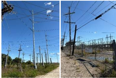
Figure 1: Required Powerline Relocations and Adjacent Entergy Substation
