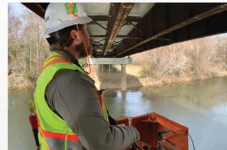
**State Aid Complex Bridge Inspections and Load Ratings (2019-2020).** AECOM provided inspection and load ratings of 88 bridges that were identified as having steel superstructures. The bridges were inspected following the same scope as the complex inspections described in the 2021-2022 cycle narrative.
