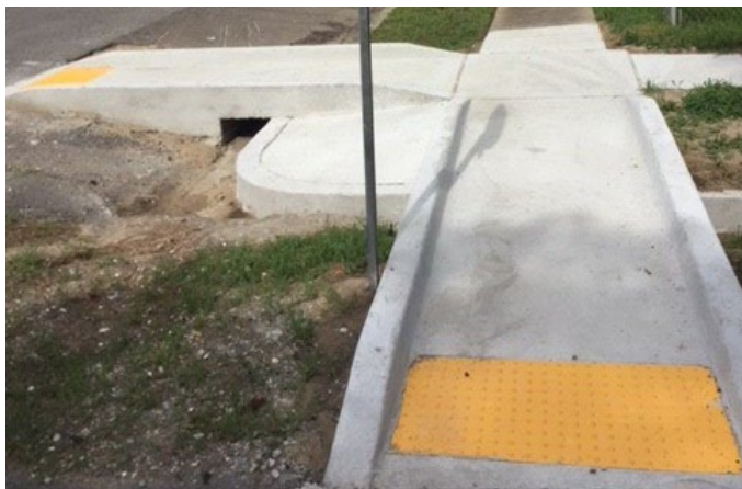
Figures: Implemented new sidewalk, crosswalk, ADA ramps and pedestrian enhancements
