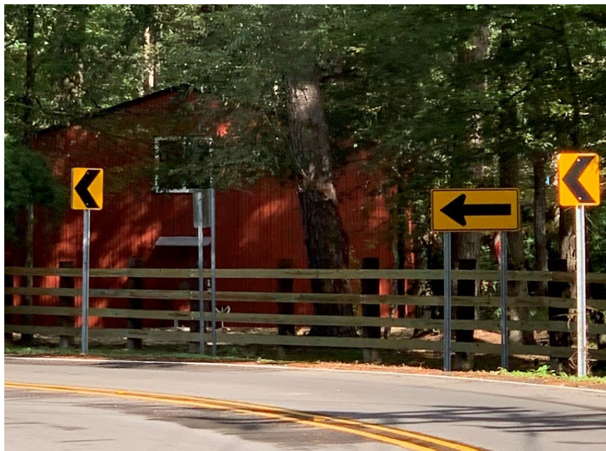
Figure: Implemented New Signage, Striping and Pavement Markers for Curves
