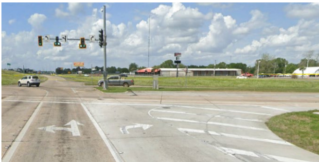
Figure: Implemented low-cost improvement to remove channelized right turn lane @ Gloria Switch Rd
