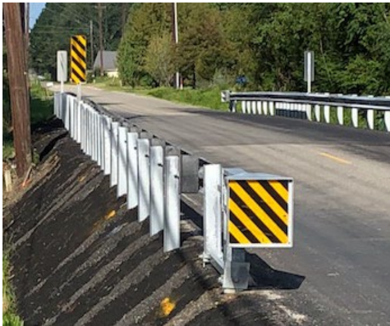
Figure: Installation of LADOTD compliant guardrails
