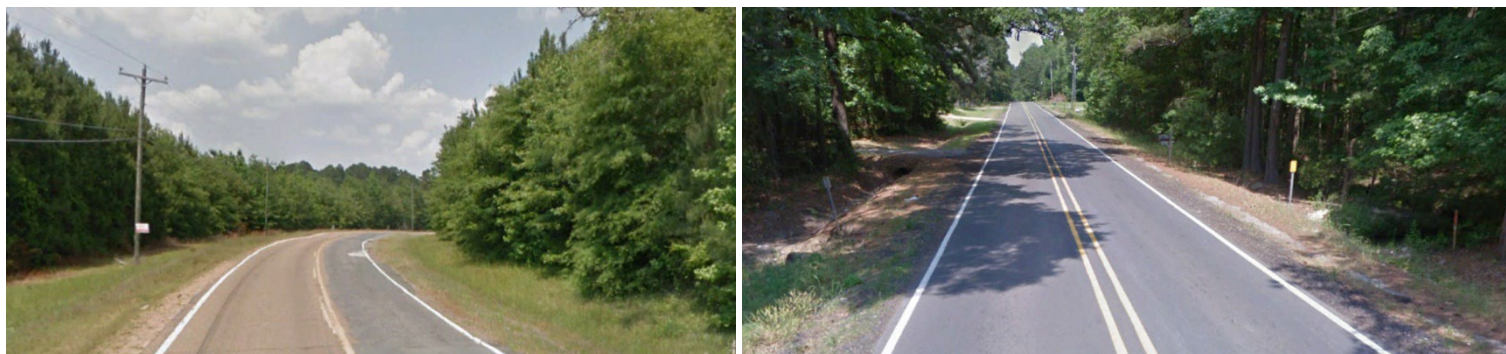
Existing Conditions of LA 117 Showing Narrow Shoulders and Example of Horizontal and Vertical Geometry
