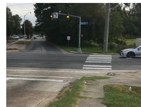
Figure: Photo taken during RSA showing condition of sidewalk and curb ramps
