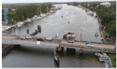
Figure: Existing Swing Span Steel Bridge Over Tchefuncte River
