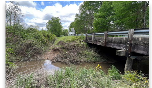
Looking east showing bridge, channel and ditch Site Visit - (4/2/2025)
