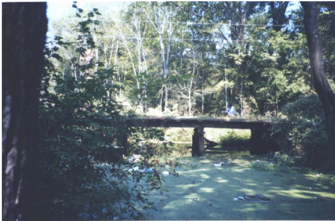
PHOTOGRAPH 6: BRIDGE DOWNSTREAM SIDE, LOOKING FROM CHANNEL BANK
