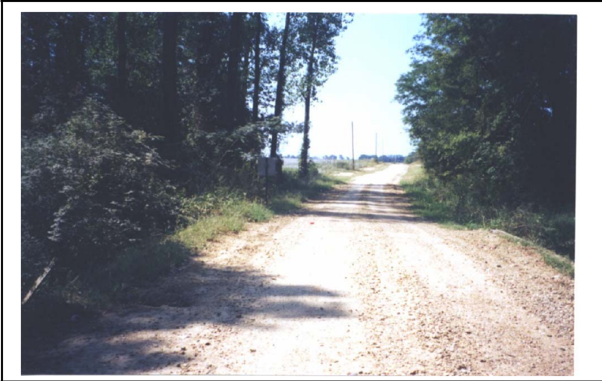
PHOTOGRAPH 1: ROADWAY VIEW, LOOKING WEST FROM BRIDGE
