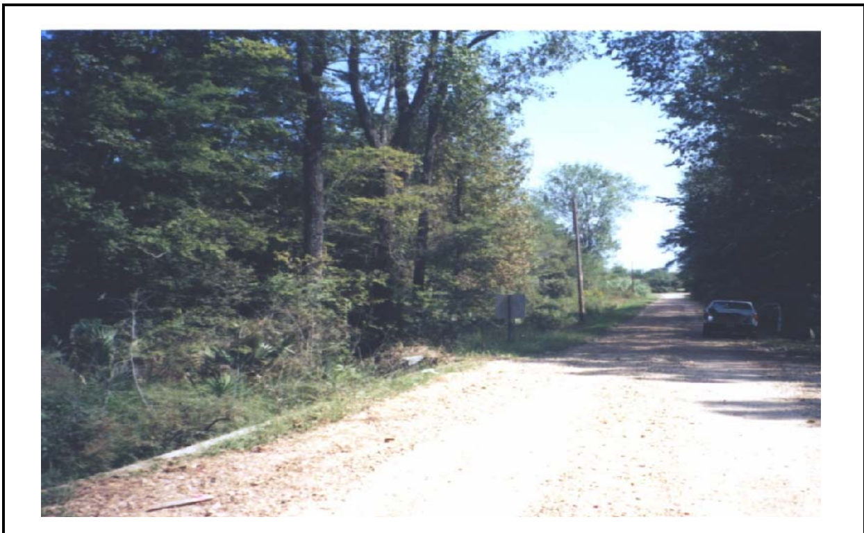
PHOTOGRAPH 2: ROADWAY VIEW, LOOKING EAST FROM BRIDGE
