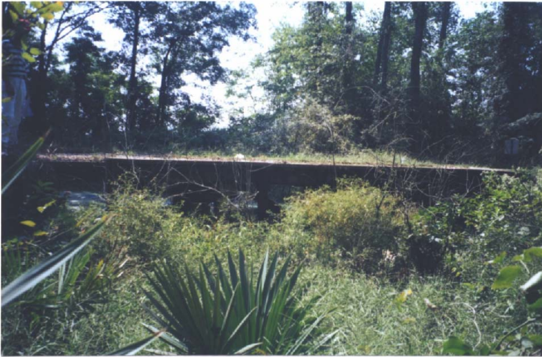
PHOTOGRAPH 5: BRIDGE UPSTREAM SIDE, LOOKING FROM CHANNEL BANK
