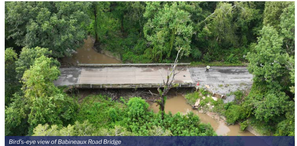
Bird's-eye view of Babineaux Road Bridge
