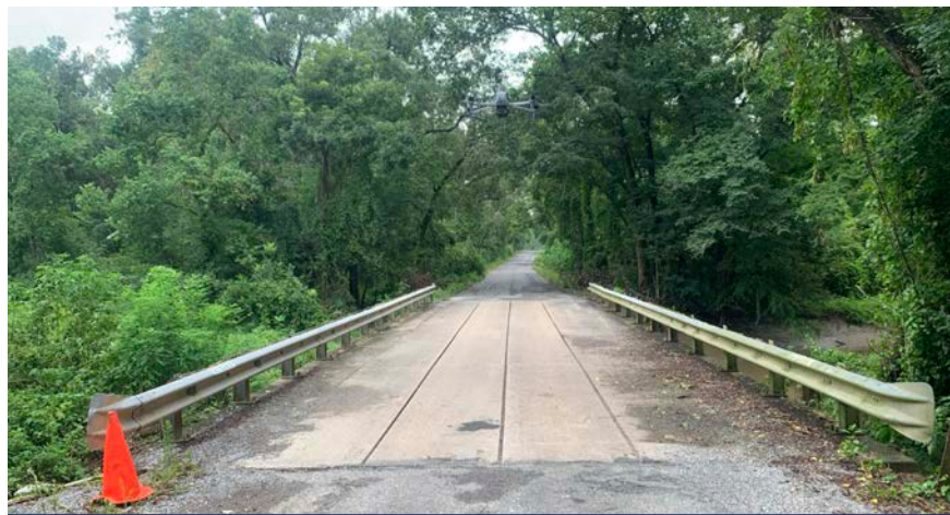
Street view of Babineaux Road Bridge
