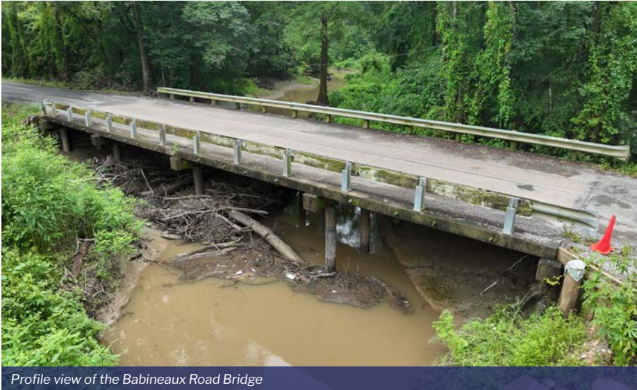
Profile view of the Babineaux Road Bridge
