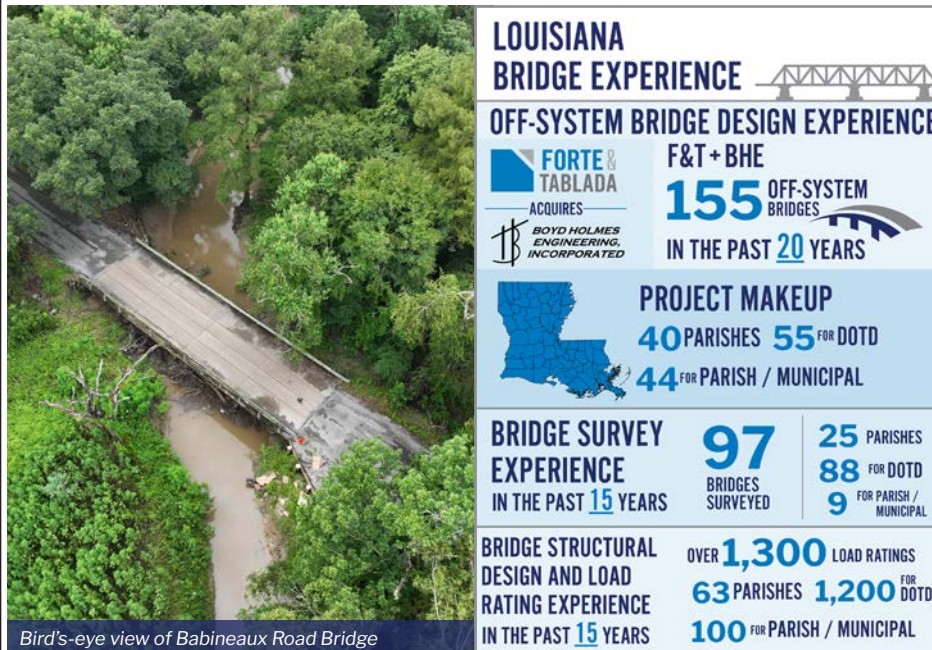
Bird's-eye view of Babineaux Road Bridge
