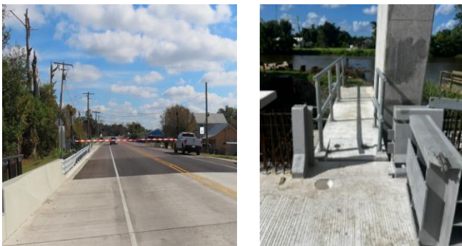
H&H provided pedestrian and bridge traffic gates CE&I Services for Company Canal in Bourg, LA for LADOTD
