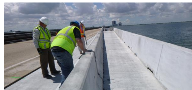
H&H is providing CE&I Services including bridge lighting and traffic signal systems for the Causeway Bridge in New Orleans, LA
