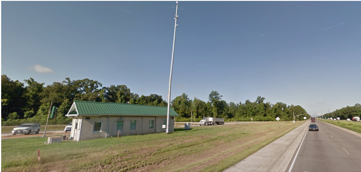
Figure 16: Weigh Station on I-12
