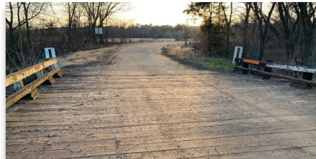
Begin bridge side of Hosston River Bridge/ Kelly Bayou - showing existing horizontal geometry without superelevation
