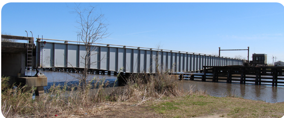
This 1965 swing bridge features what is known as a bobtail swing span due to span arms that are different lengths on either side of the pivot pier (Little Prairie Bridge, Bridge Recall No. 009690).
