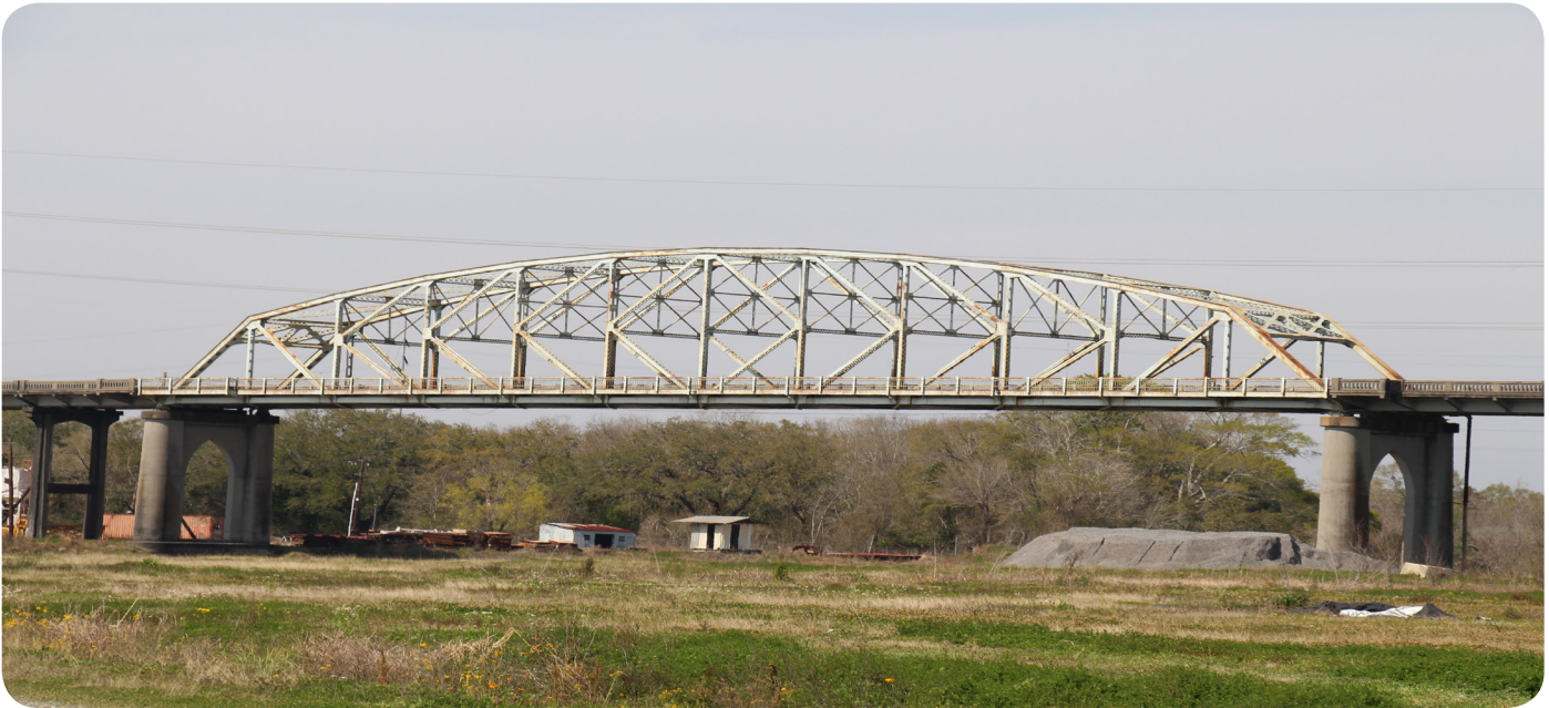
K-truss through bridge (Charenton Bridge, Bridge Recall No. 008970).
