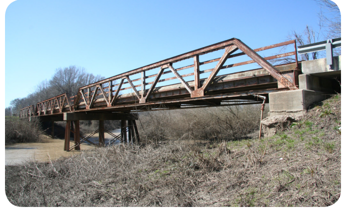
Warren pony truss bridge (Tensas River Bridge, Bridge Recall No. 400345).
