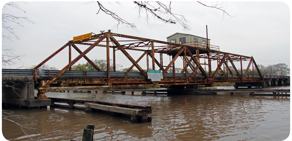
The turning mechanism of this 1960 through truss swing span is situated on a pivot pier and the operator's house is centered above the roadway (Bayou Tigre Bridge, Bridge Recall No. 010130).
