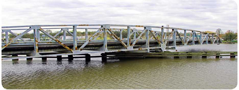
Pony truss swing bridge in motion (Kerner Ferry Bayou Bridge, Bridge Recall No. 000810).
