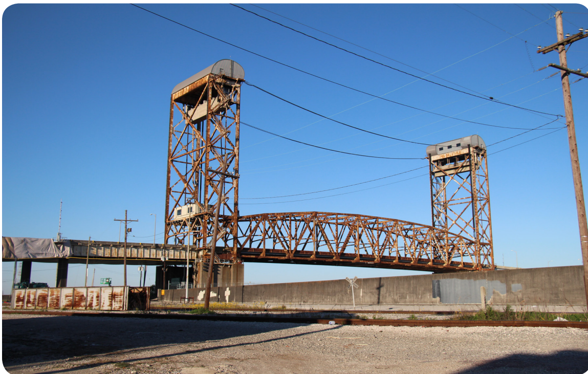
Tower drive vertical lift bridge with independent towers. Operational machinery is located in shed-type structures on top of each tower (Judge Seeber Bridge, Bridge Recall No. 020375).
