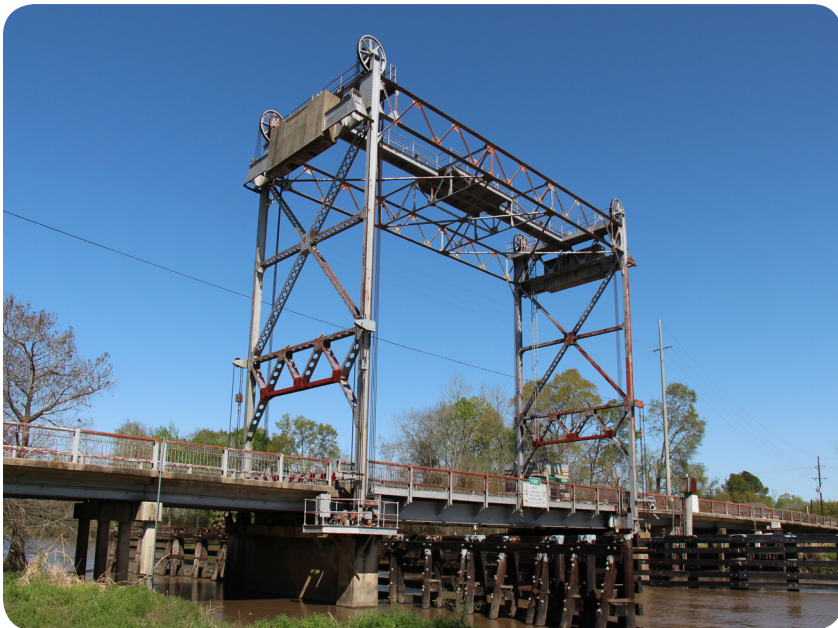
Tower drive vertical lift bridge with connected tower and drive machinery on the platform between the towers (Vermilion River Bridge at Perry, Bridge Recall No. 009680).
