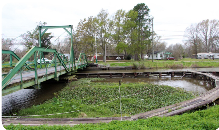
Cable-stayed swing bridge with its characteristic system of ropes and pulleys that operate the bridge (Terrebonne Parish Road No. 293 Bridge, Bridge Recall No. 200852).
