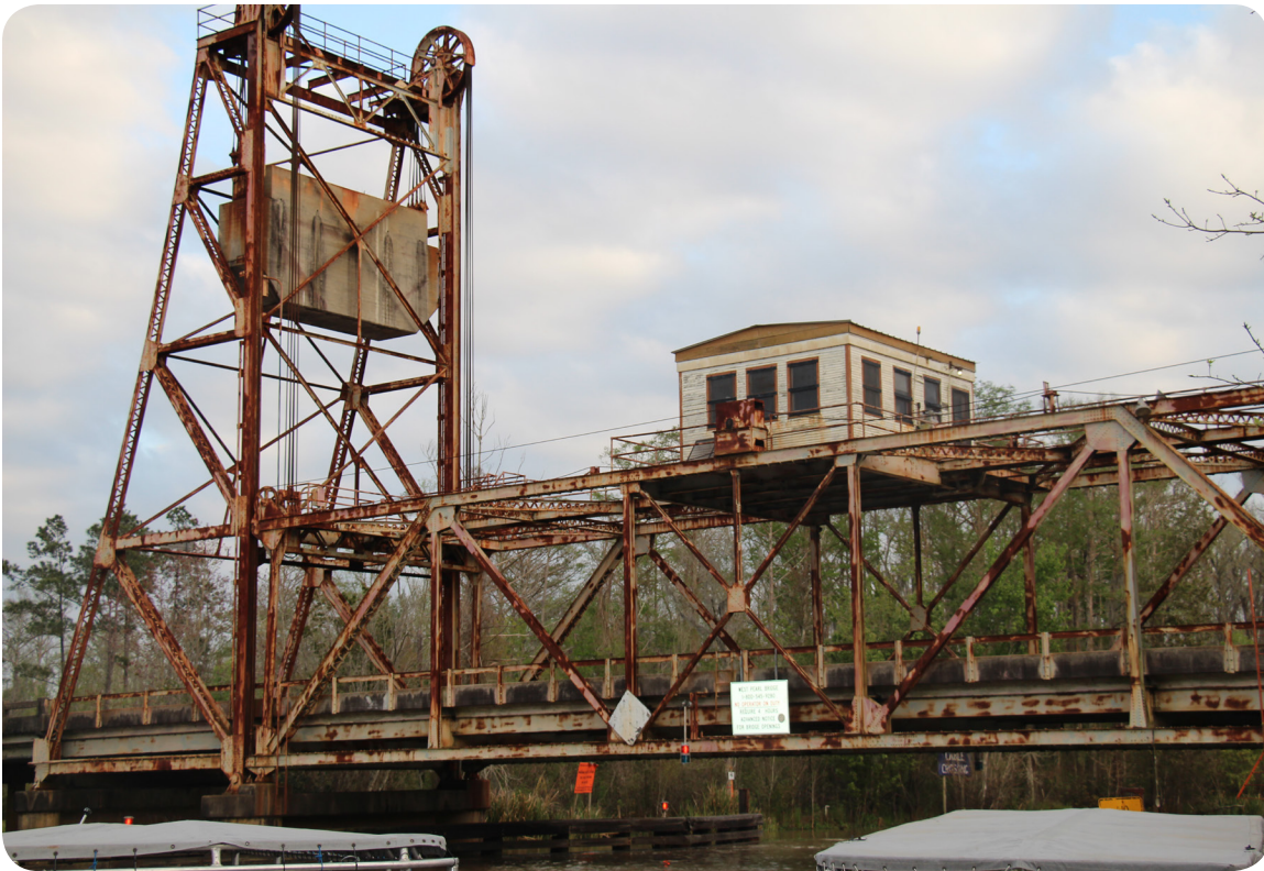
Span drive vertical lift bridge. Operational machinery is located on top of the upper chords (West Pearl River Bridge, Bridge Recall No. 058710).
