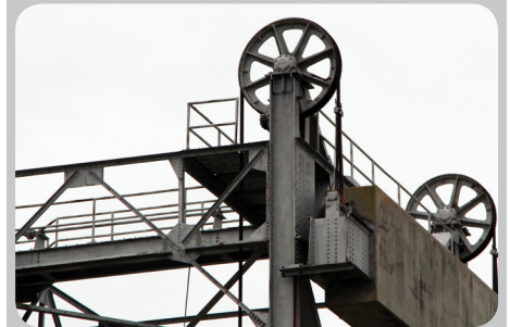
Sheaves and operating ropes/cables on the Sarah Road - Bayou Petit Caillou Bridge (Bridge Recall No. 003480).
