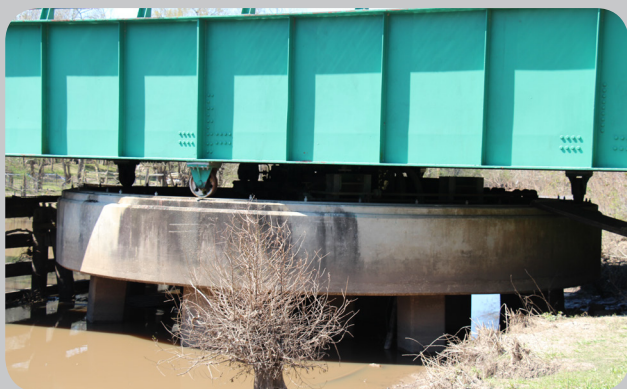
Center-bearing mechanism (Bayou Teche at Morbihan Bridge, Bridge Recall No. 006200).
