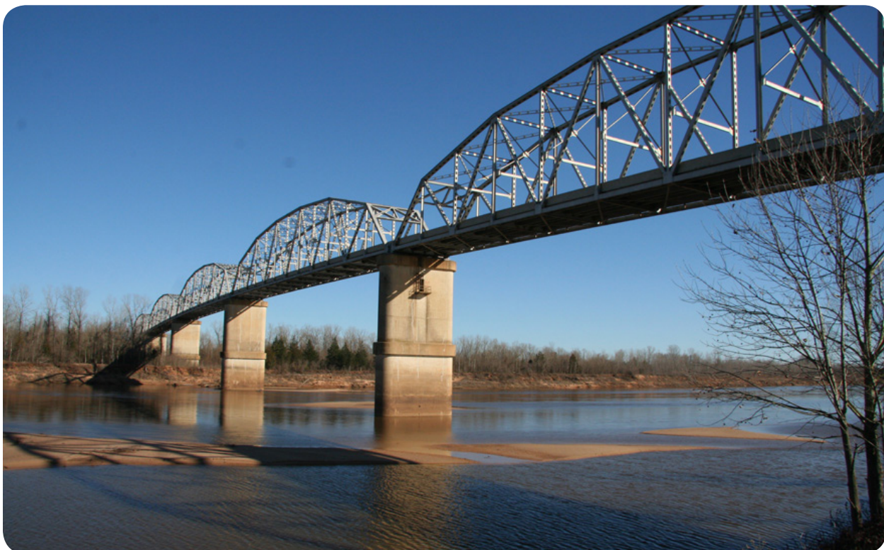
Warren through truss bridge (Miller's Bluff Bridge, Bridge Recall No. 012548).
