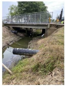
storm drain outfall pipes, and storm drainpipe tie-ins to proposed box culverts. Furthermore, Fenstermaker is performing scour analyses and providing recommendations for channel erosion protection measures. All data is analyzed using HEC-HMS, HEC-RAS, and the **LADOTD HYDRWN** software.
