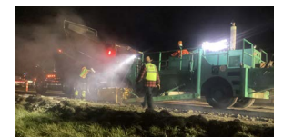
US 90 construction operations: slab jacking (left) and asphalt overlay (right).
