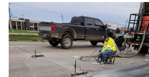
US 90 construction operations: slab jacking (left) and asphalt overlay (right).
