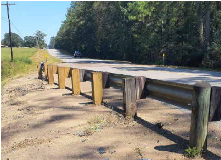
LA 10 guardrail repair
