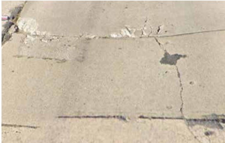
Concrete cracking on LA 511
