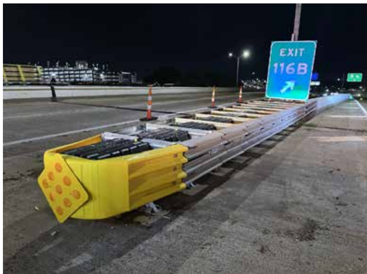
Crash attenuator after repairs
