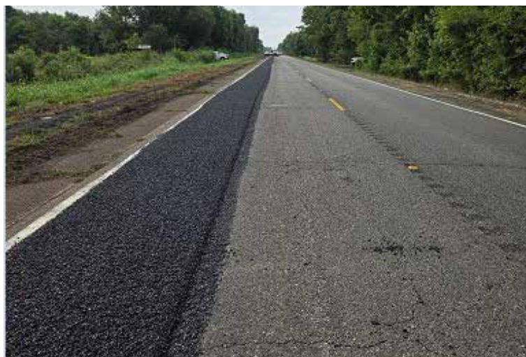
Rut busting project on the northbound side of U.S. 71
