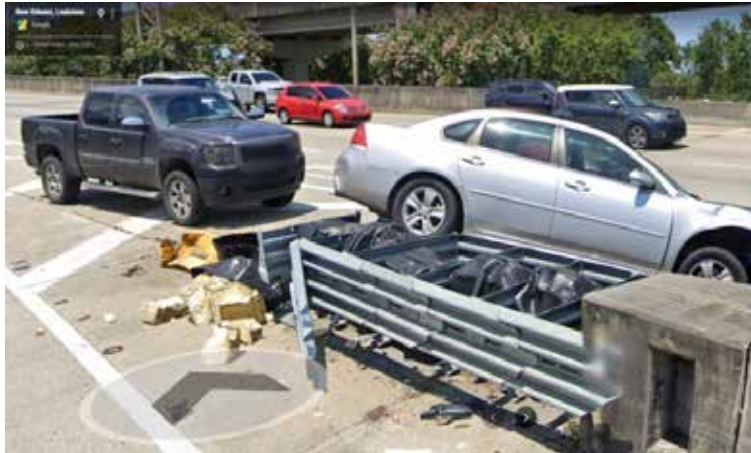
A damaged impact attenuator
