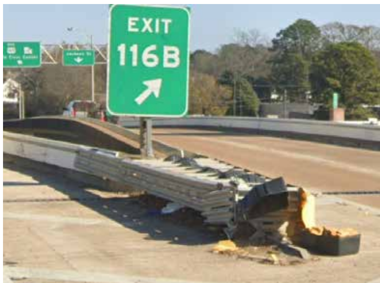
Damaged crash attenuator in Ouachita Parish
