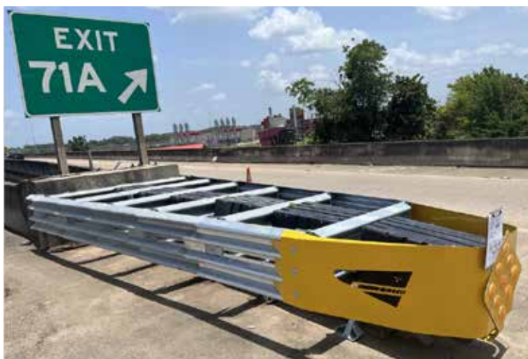
Repaired impact attenuator in Rapides Parish
