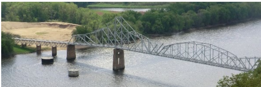
For the Blackhawk Bridge over the Mississippi River in Iowa, HDR designed a dolphin system to improve the resilience for this truss bridge.
