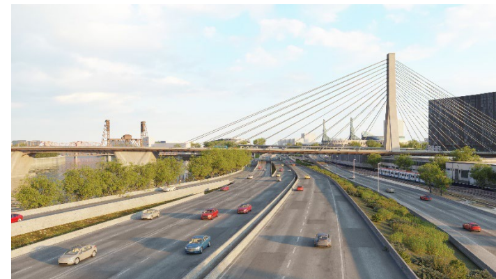
The inverted-Y-shaped tower of the cable-stayed bridge is located east of Interstate-5 and a UPRR mainline. Doing so avoids up to eight feet of seismically induced lateral displacements that a conventional span arrangement would experience towards the Willamette River.
