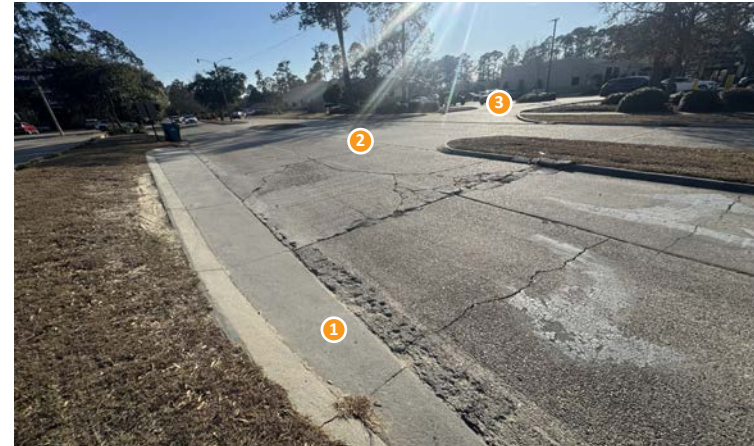
Figure 1. Our team has conducted a site visit along Lakewood Drive to evaluate key considerations for sidewalk construction and concrete panel replacement. Experience delivering similar neighborhood and residential projects allows our team to anticipate challenges and implement proactive solutions that support successful project delivery.
