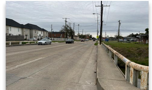
Looking north showing sidewalk and utilities Site Visit (3/4/2024)
