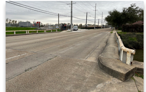
Looking south showing bridge, transmission line and detention basin - Site Visit (3/4/2024)
