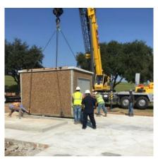
Arcadis provided CEI services for the US 190 ITS Deployment project in West Baton Rouge, Pointe Coupee, and St. Landry parishes. This project consisted of the installation of approximately 225,000 feet of fiber optic cable and conduit, the installation of two communication HUB buildings, and the interconnection of four signalized intersections onto the state communications network. The project had a construction cost of \$2.3 million.
