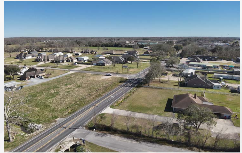
This image shows a constructed project completed by NSI which included similar tasks as this contract.
