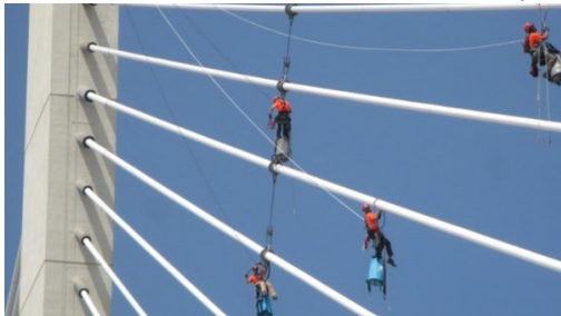
➤ Rope Access Inspection of US 82 Cable Stay over Mississippi River, Greenville, MS
