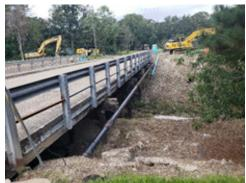
Both bridges were located in a FEMA flood plain and the 100 year design water surface could not be raised
