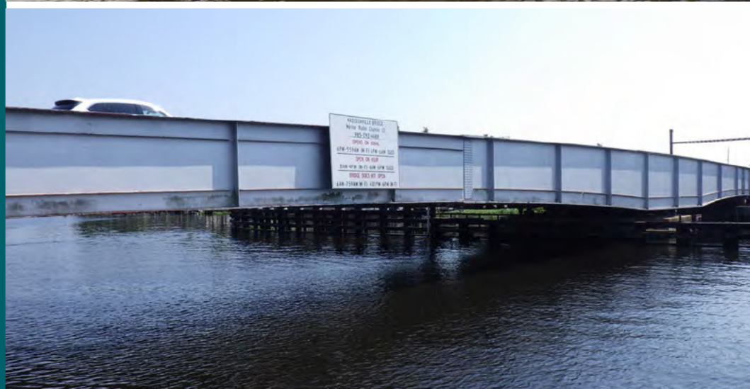
Bridge 059482 - LA 22 over Tchefuncte River (Steel Girder Swing Span Bridge)
