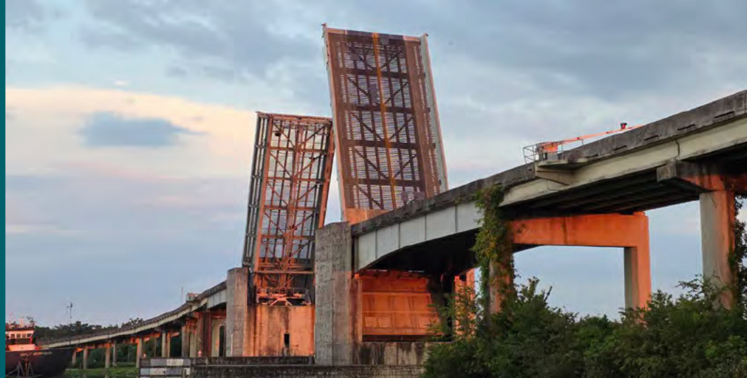
Bridge 003412 - LA 315 over Bayou Dularge (Steel Girder Bascule Bridge)
