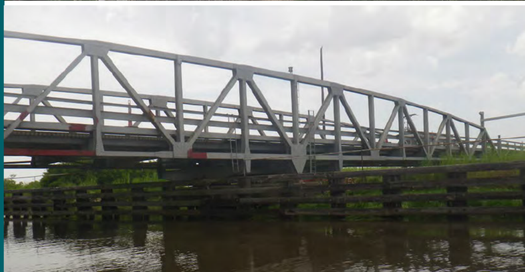
Bridge 033730 - LA 82 over Superior Canal (Steel Pony Truss Swing Span Bridge)
