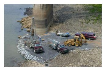
As part of the project, Ardaman developed a full slope stabilization design and construction remediation strategy and a monitoring program for the bluff instability and ground movements affecting the existing I-20 Mississippi River Bridge.
