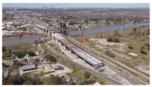
The project is a P3 project which consists of replacing the existing Belle Chasse Tunnel and Judge Perez Lift Bridge at the Algiers Canal. Proposed improvements included a four-lane fixed height bridge with pedestrian and bicycle accommodations. The project alignment is from Engineers Road, about 2,000 feet northwest of the Intercoastal Canal to some 2,300 feet southeast of the canal between the existing Belle Chasse tunnel and the lift span bridge.
