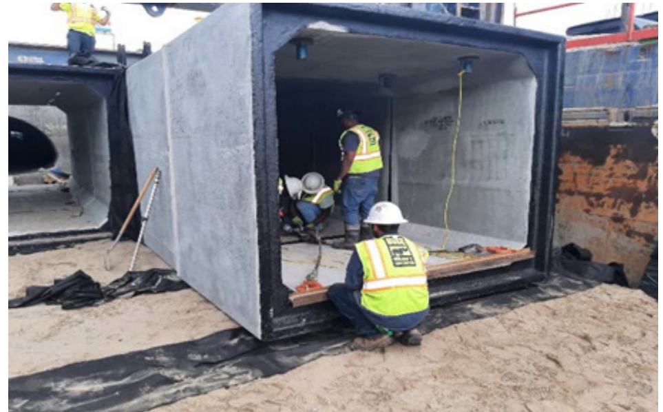
Precast Box Culvert Installation on I-10/Loyola Interchange Improvements
