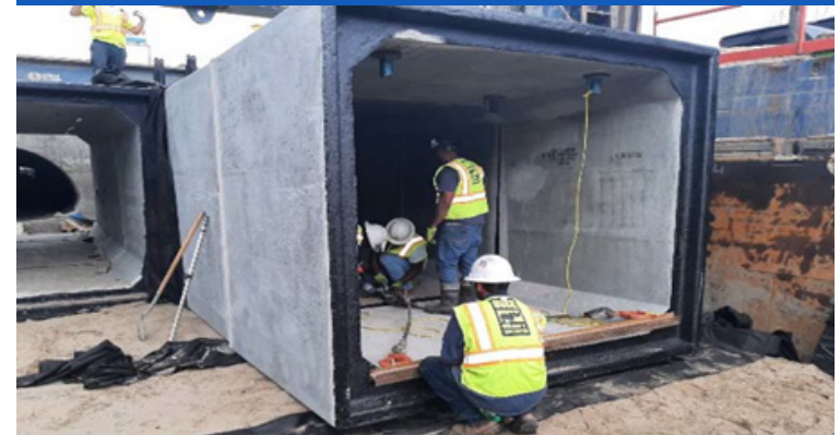
GEC oversaw installation of 625' of double barrel precast box culvert units to Canal 13. This included subsurface drainage tie-in and the construction of the westbound on/off ramps over it.
