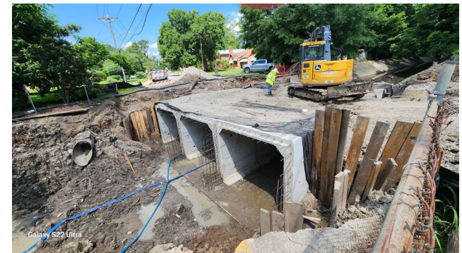
GEC oversaw installation of a triple barrel box culvert in Baton Rouge.
