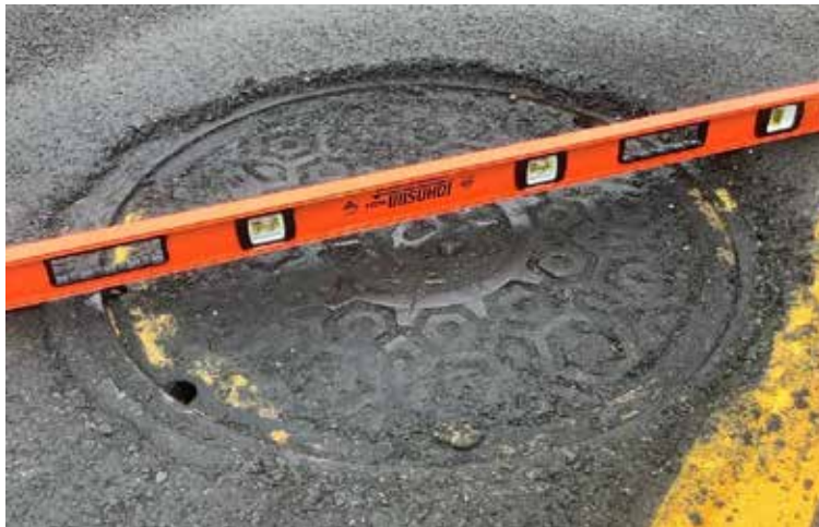
Measuring hot mix at a manhole cover
