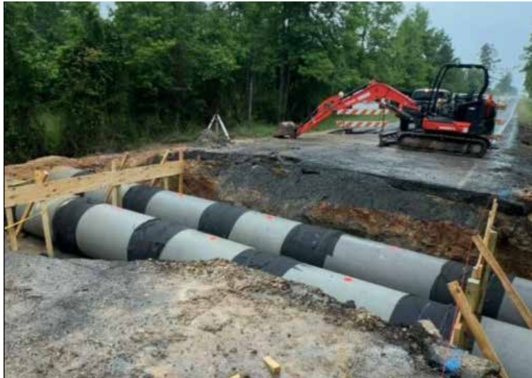
Cross drain replacement on LA 113 in Beauregard Parish
