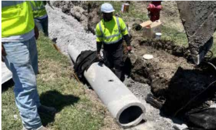
Installation of drain pipe on LA 56
