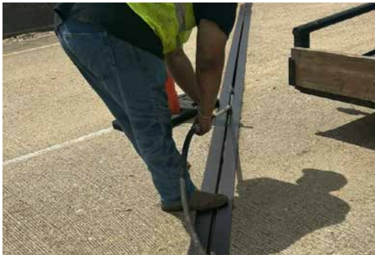
Sealing a bridge joint
