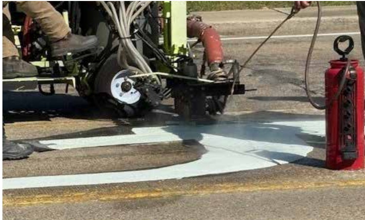
Thermoplastic striping to increase roadway visibility
